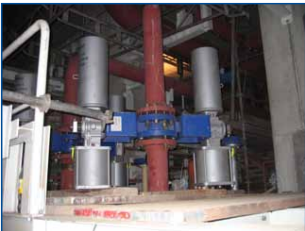
ESD turbine trip
